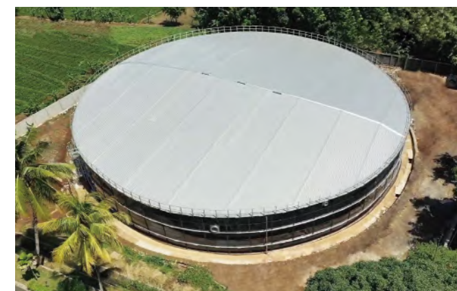
Potable Water Storage GFS tanks
