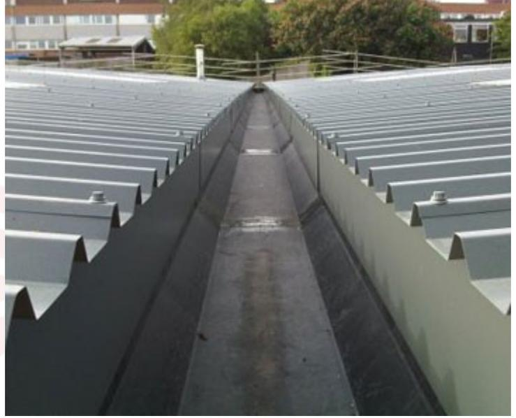
**WATER DRAINAGE CHANNELS ON STEEL ROOFS**
