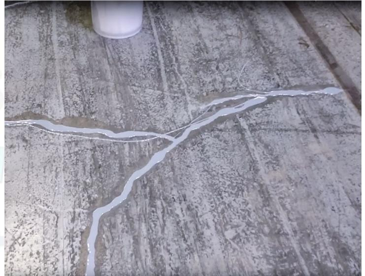
JOINTS & CRACKS REPAIR
